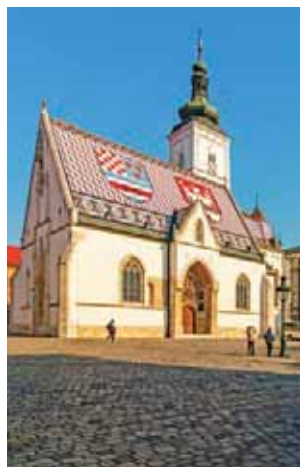
St. Mark's Church, Zagreb
