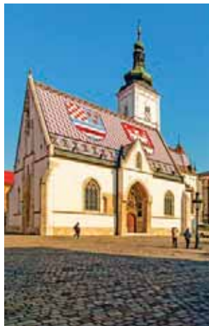
St. Mark's Church, Zagreb
