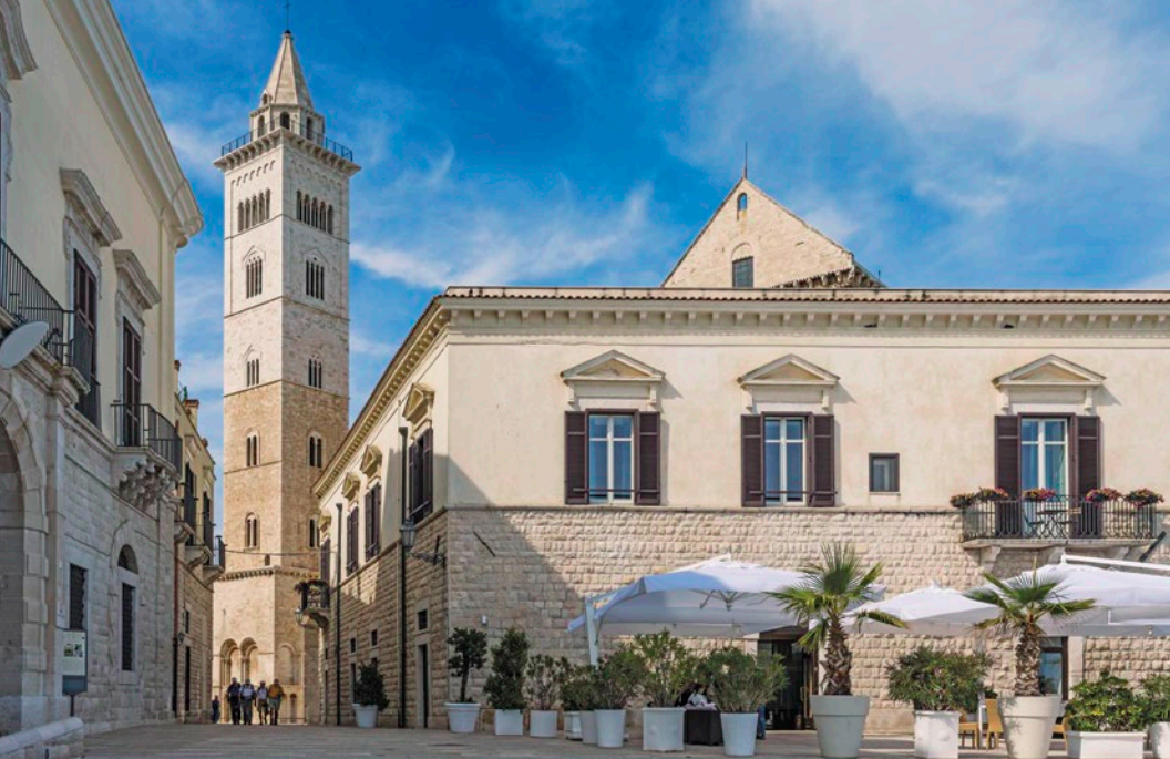
Cathedral bell tower, Trani
