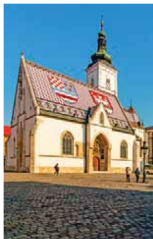
St. Mark's Church, Zagreb
